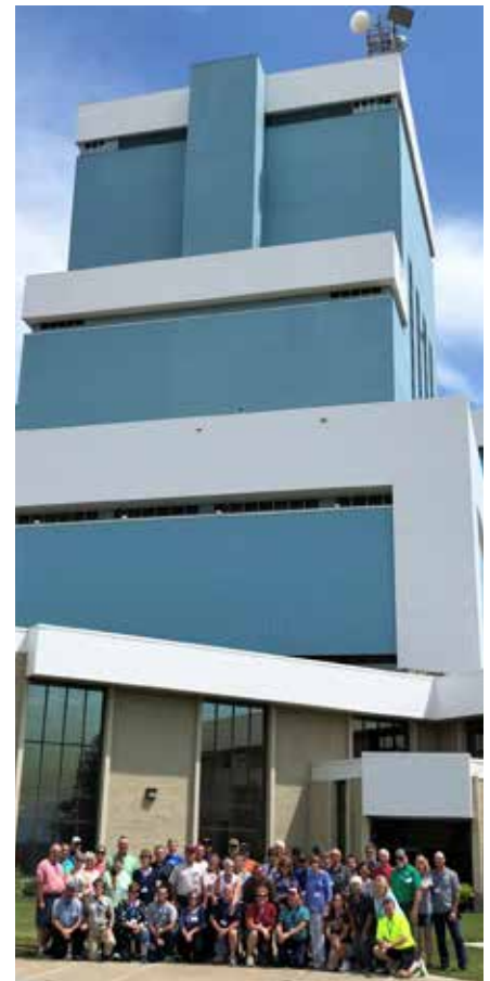
Energy Trail Tour participants pose for a group shot in front of Basin Electric Power Cooperative's 900-megawatt Antelope Valley Station, a coal-fired electric generation station.
