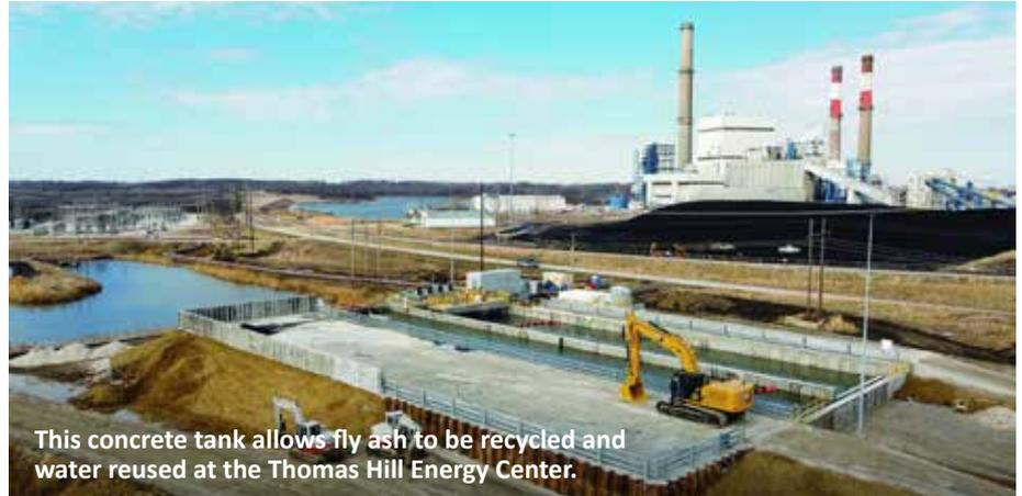
This concrete tank allows fly ash to be recycled and water reused at the Thomas Hill Energy Center.
