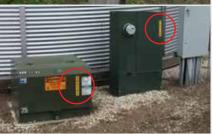
the tags are on a pole, they are usually mounted approximately 5 feet above the ground line and face a road or driveway. Ground-mounted equipment will have tags on the lid or door next to other warning stickers.
