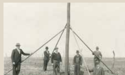
Cost to install a pole in 1940 $27.43
